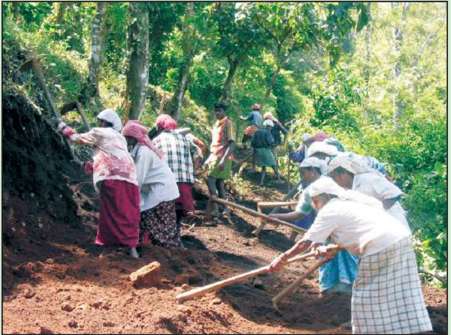
Workers at worksite in Kerala. Photo Credit: Dr. Jyothi Krishnan
