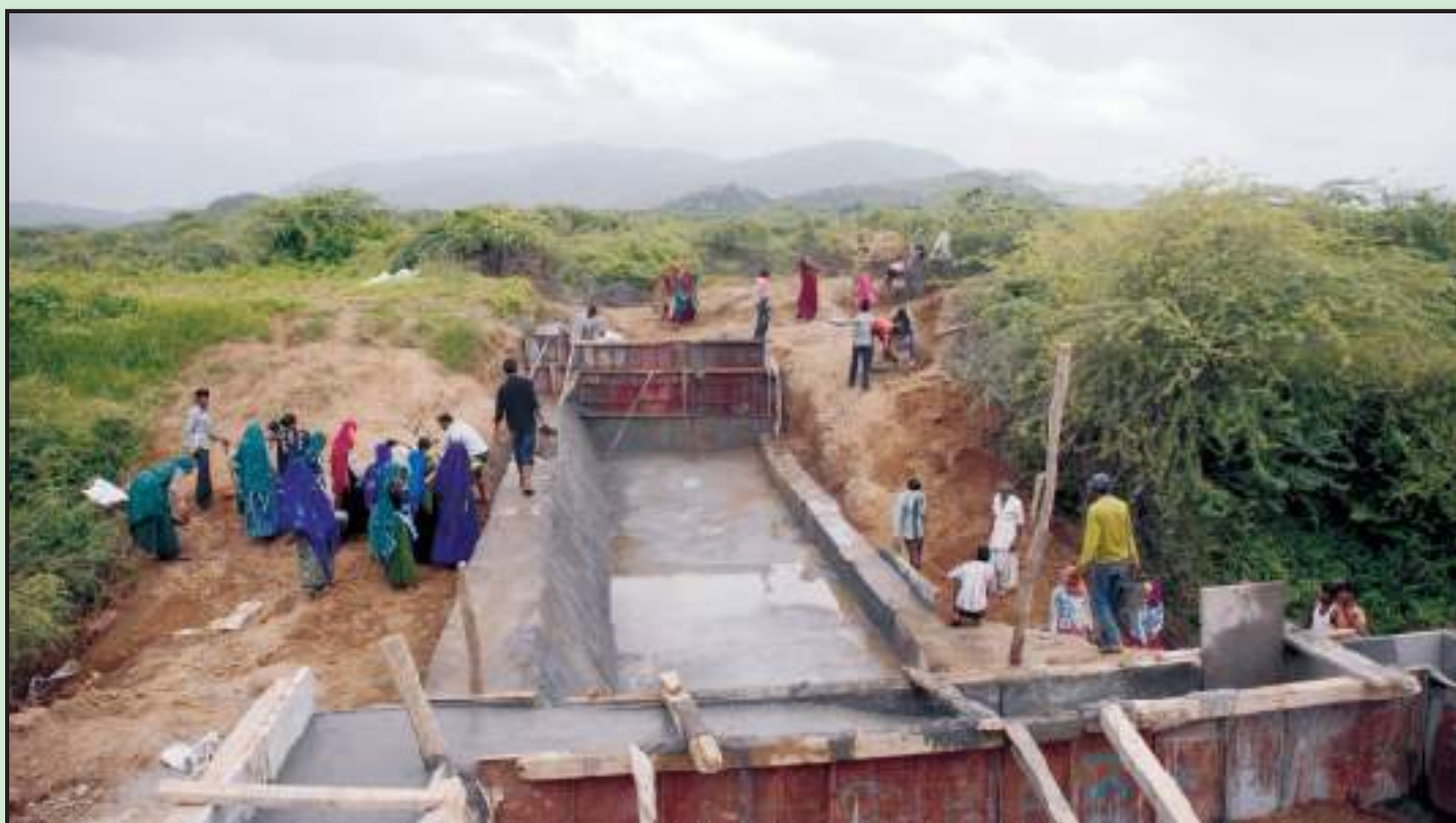
Check Dam Construction Under Mgnrega in Village Nichala Bandh, Block Amirgarh, District Banaskantha, Gujarat
